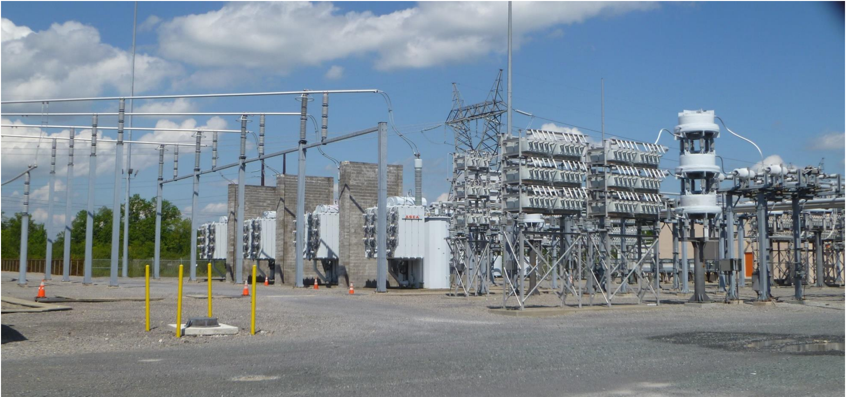
FIGURE A.3: Capacitor II
