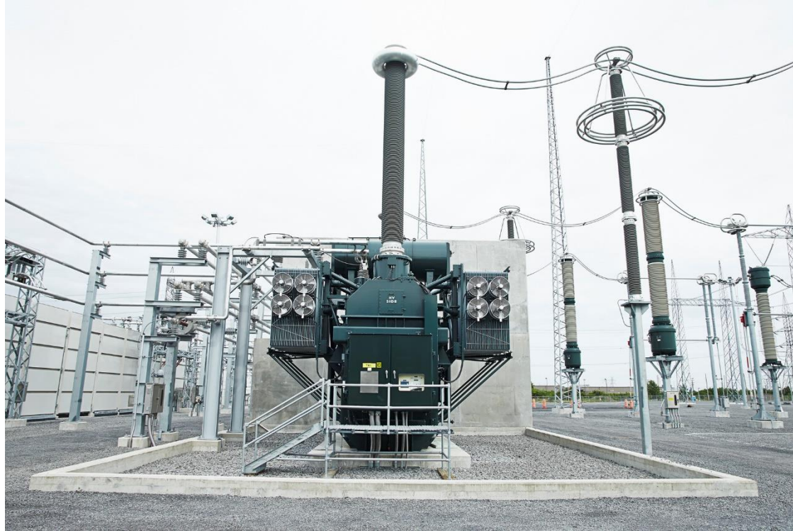
FIGURE A.5: Static VAR Compensator
