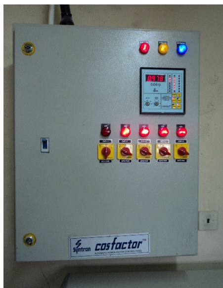
Figure 4.9 Example of a PF Capacitor Bank on a motor load
