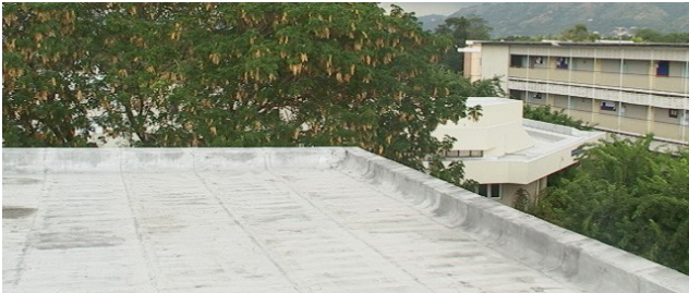
Figure 4.3 Example of coated roof in Kingston, Jamaica
