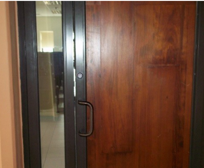
Figure 4.1 Example of air gap between door and mull post
