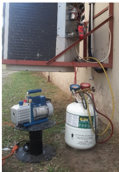
Figure 4.5 Refrigerant in an AC unit being changed
