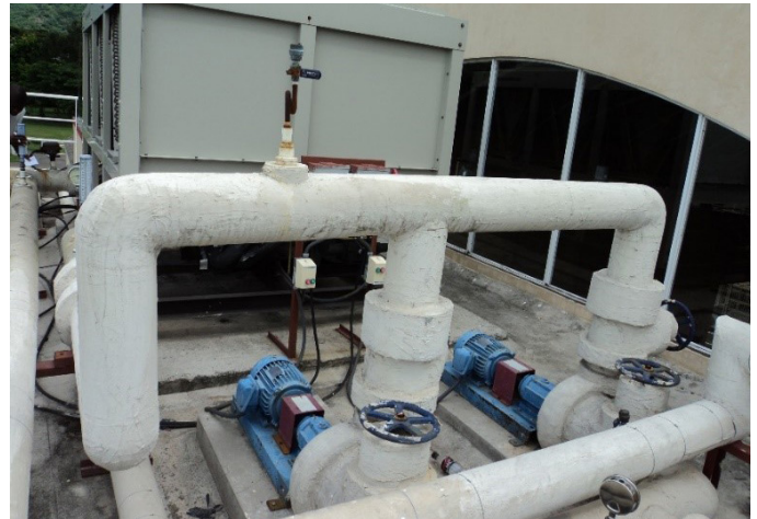
Figure 4.4 Example of some insulated chilled lines
